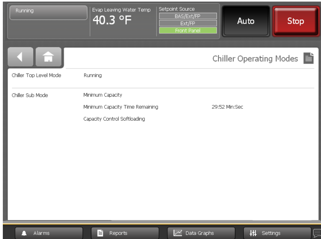
Figure 12. Chiller Operating Modes screen for Simplex chillers
