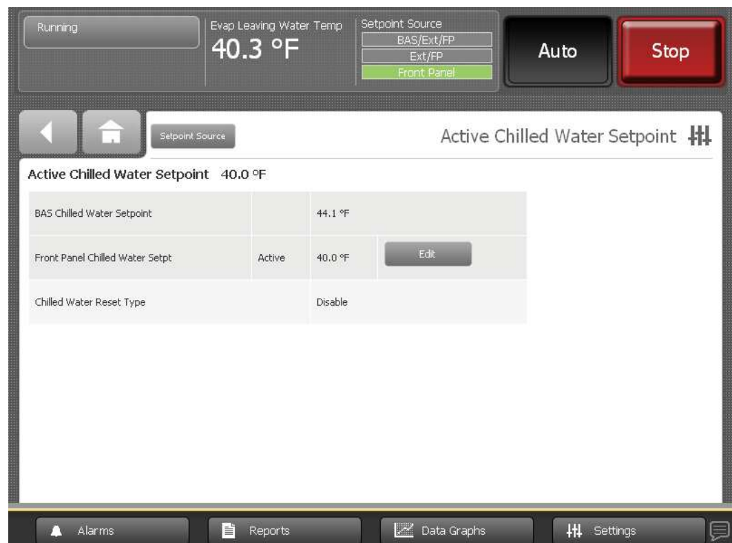
Figure 26. Changing the setpoint source from an arbitrated setpoint screen
