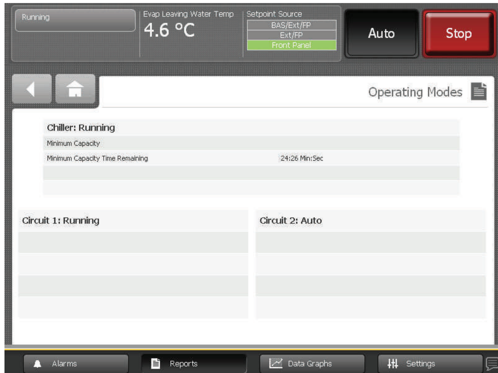
Figure 13. Chiller Operating Modes screen for Duplex chillers
